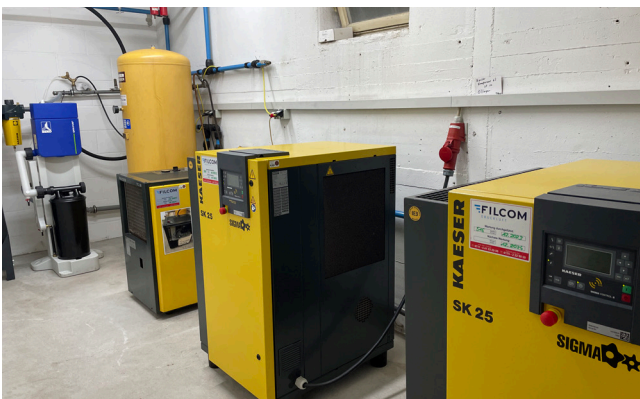
The new compressed air station could be accommodated in a technical room. Picture source: Speick Naturkosmetik
