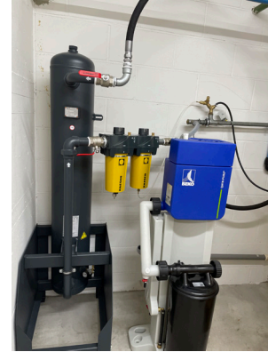
Oil-water separator QWIK-PURE for condensate treatment Picture source: Speick Naturkosmetik
