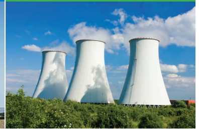
POWER PLANTS & ENERGY
