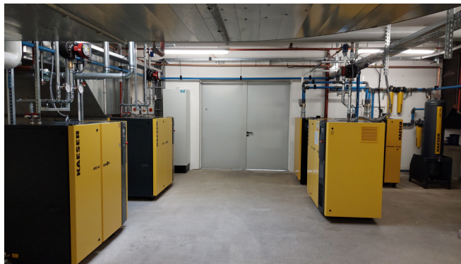
View of the KAESER compressed air station at Gebr. Schwarz GmbH Picture source: Gebr. Schwarz GmbH
